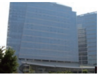
Guangzhou FA Center MITSUBISHI ELECTRIC AUTOMATION (CHINA)LTD.
