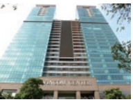
Ho Chi Minh FA Center MITSUBISHI ELECTRIC VIETNAM COMPANY LIMITED
