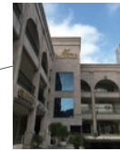
Mexico Monterrey FA Center Monterrey Office, Mitsubishi Electric Automation, Inc.
