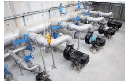
Sewage treatment plant
