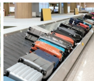
Airport baggage conveyor
