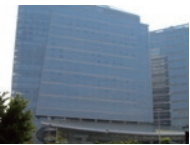
Guangzhou FA Center MITSUBISHI ELECTRIC AUTOMATION (CHINA)LTD.
