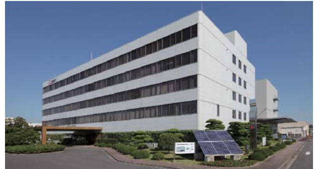
Mitsubishi Electric Fukuyama Works
